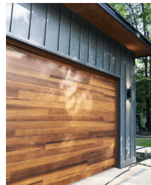
Overhead Garage Doors
