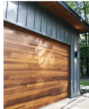
Overhead Garage Doors
